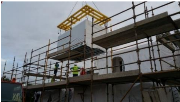
Figure 3: Module being lifted into place using a lifting frame
